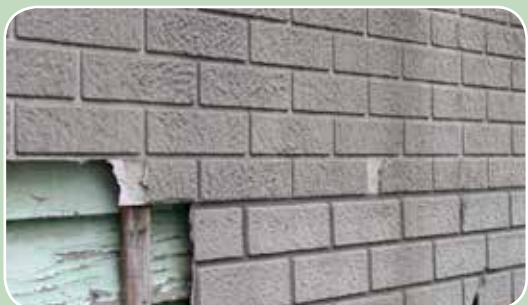
Asbestos cement 'brick' cladding
